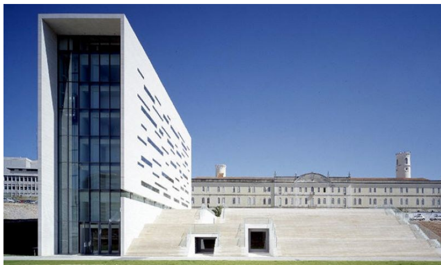
Rectorate building of NOVA University of Lisbon
